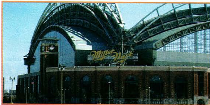
PLAY BALL Hunzinger Construction Co. built Milwaukee County Stadium, and later built its replacement, Miller Park.
