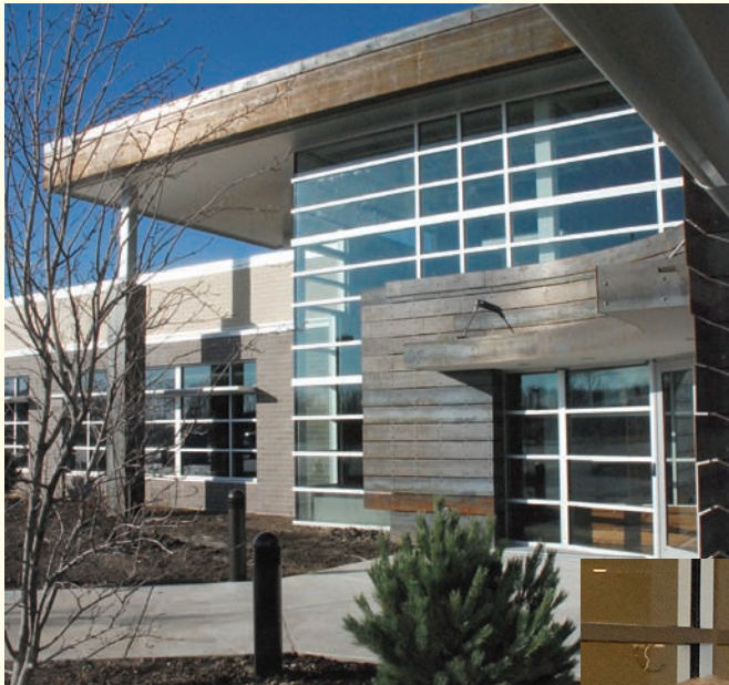
The exterior of the building includes recycled building materials, weathering Cor-ten steel, and drought-tolerant native species landscaping.
